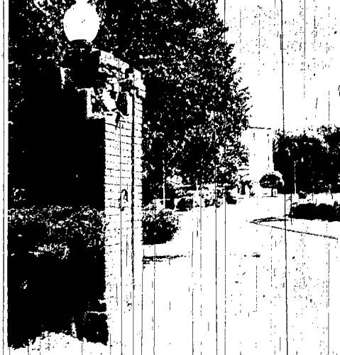
A LANDMARK on the Wayne State campus for four decades soon will be moved to a new site. The brick portals (one pictured above) at what now is the main exit on Main street have begun to crumble...
